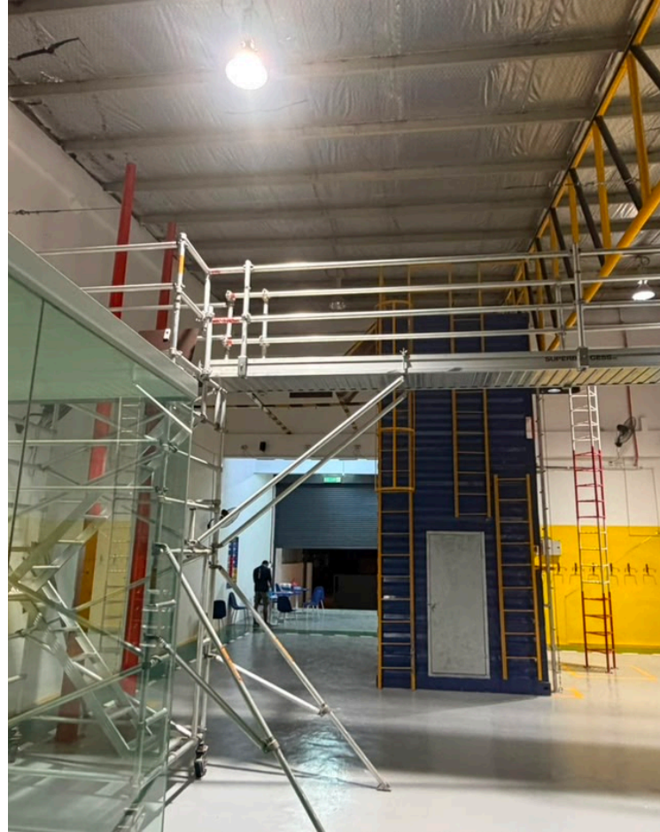
Overhead structure and suspended access area
