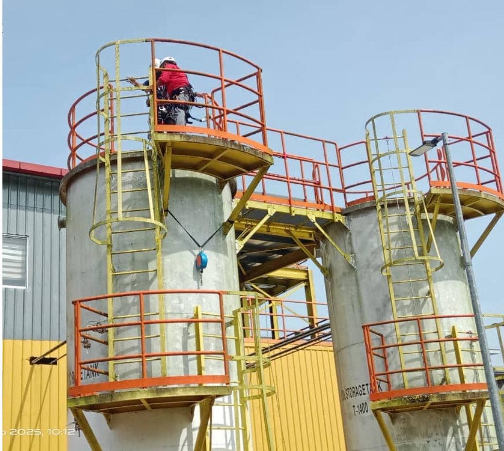
External industrial access structure
